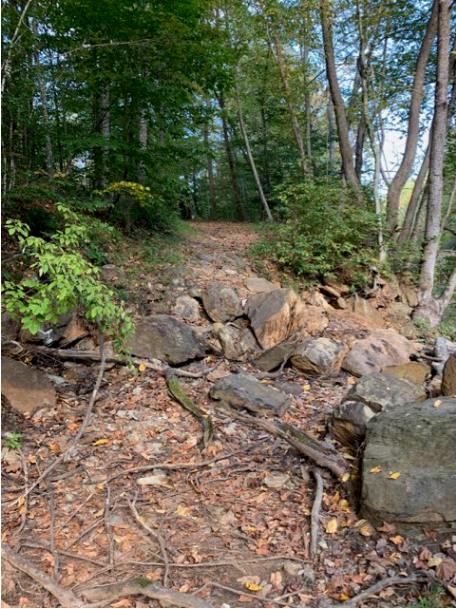
Franklin County - Erosion Exposing Large Rocks and Creating Very Uneven Ground
