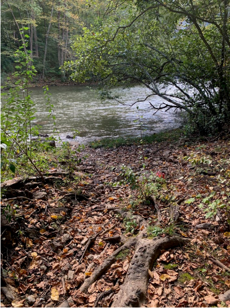
Franklin County - Severe Erosion on Launch Ramp Adjacent to River
